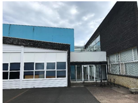
Back wall of the extension described here (blue wall at the back of the photo).
